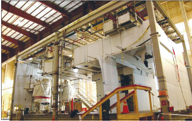
Buffer prep area in shop fabrication.
